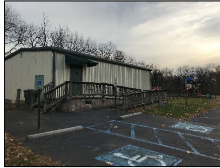
The Site Looking North
