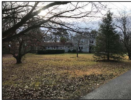
Existing Single-Family Dwelling
